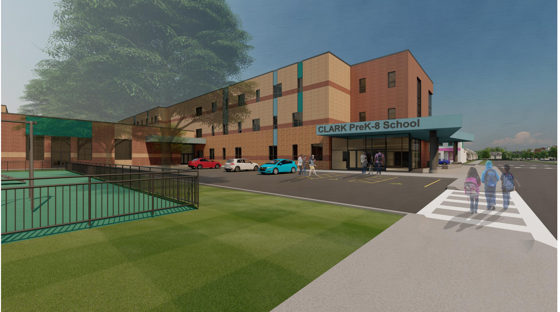
Cleveland Metropolitan School District New Clark PK-8 School Visitor Entrance – Sept. 28, 2022
